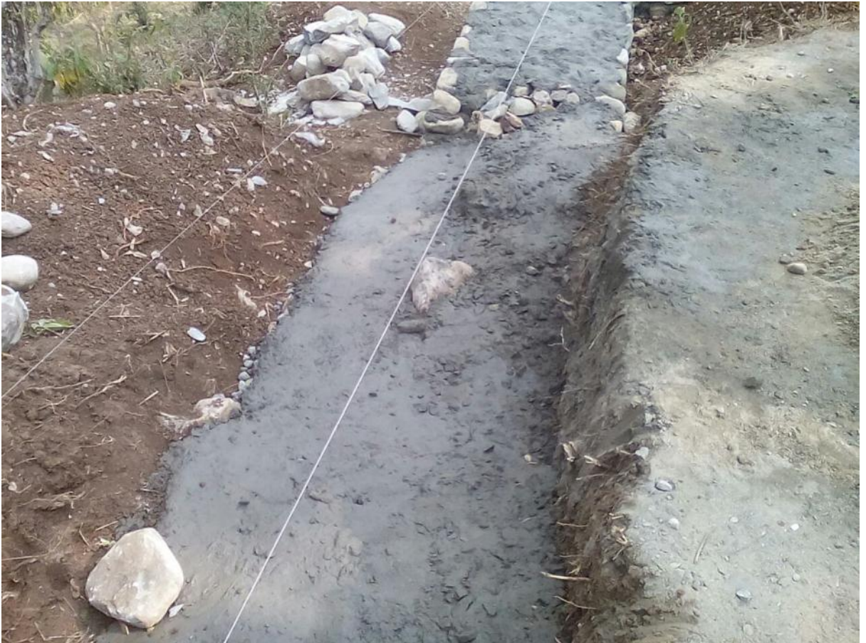
Figure 4: PCC work on foundation after stone soling
