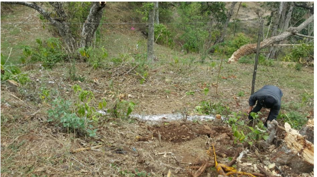
Figure 3: Land layout and side clearance by cutting tree
