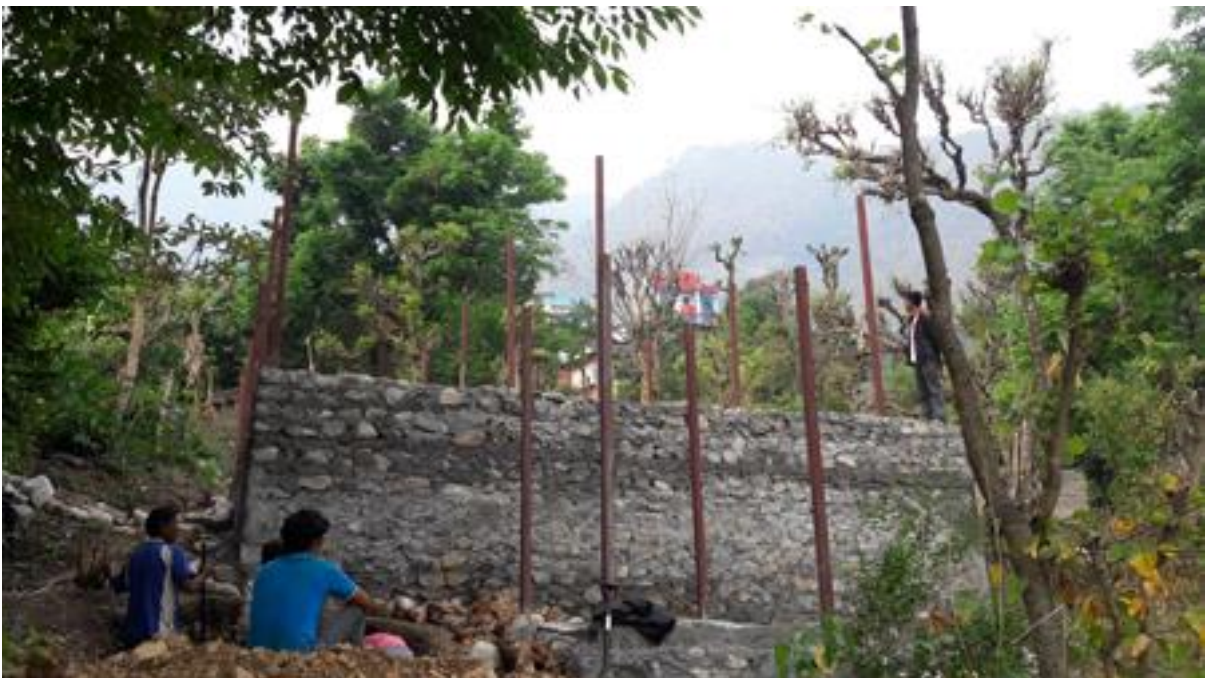
Figure 12: Toilet foundation, RCC & post erection and Septic tank excavation
