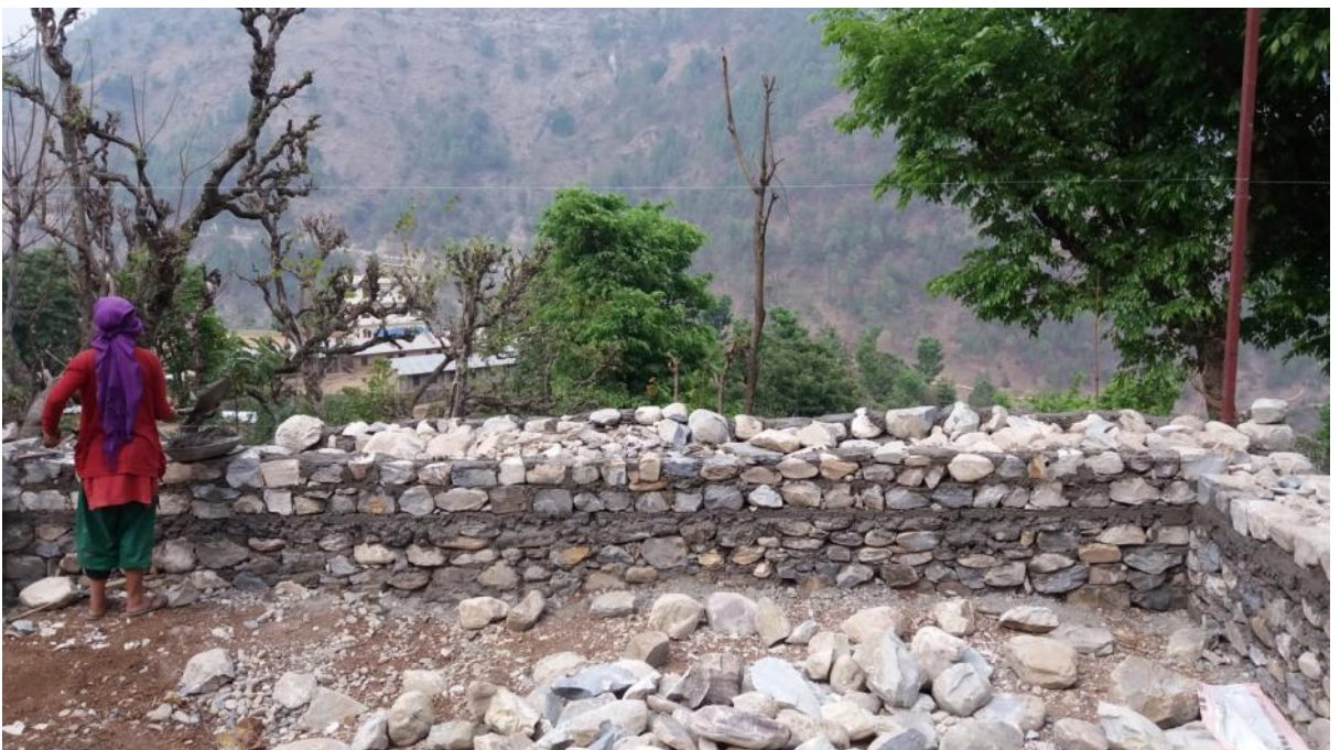
Figure 5: Stone masonry wall work for foundation and front lobby
