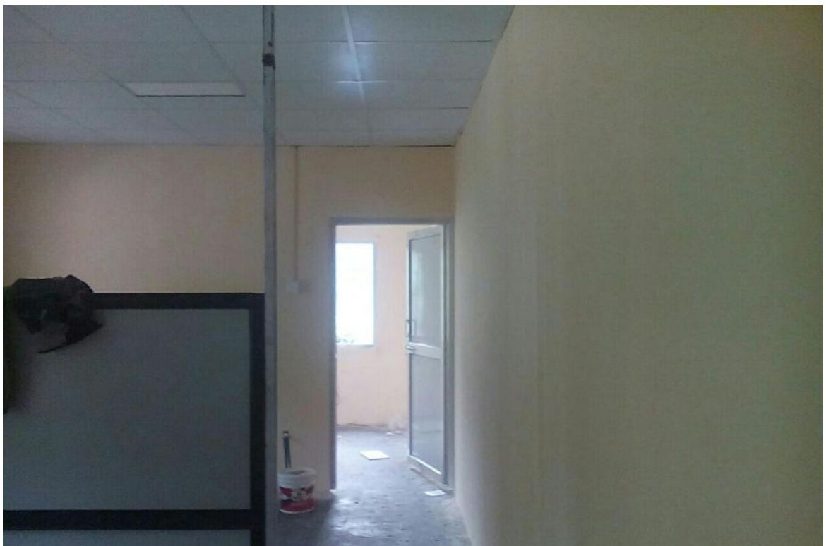
Figure 24: Completion of inner partition
