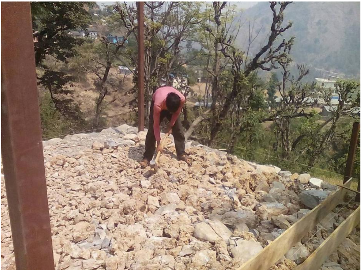
Figure 10: Compaction of soling with hammering
