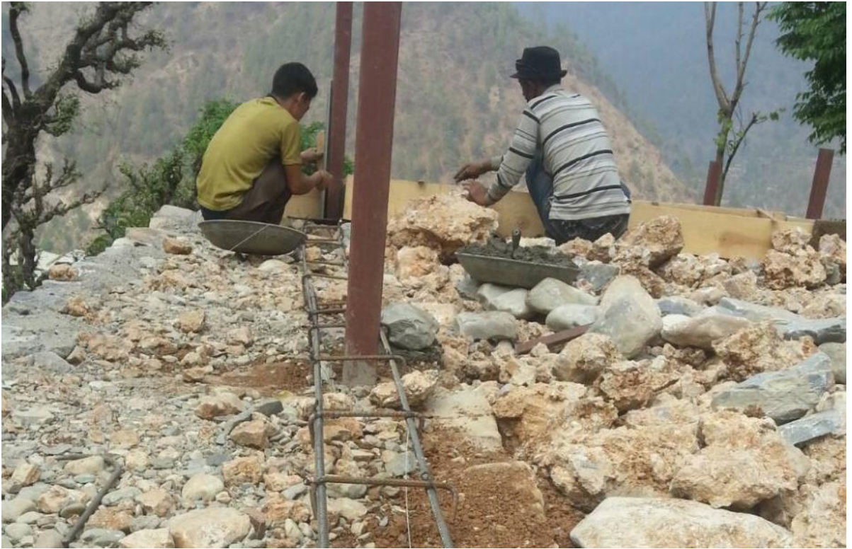
Figure 11: Reinforcement binding and formwork for RCC work
