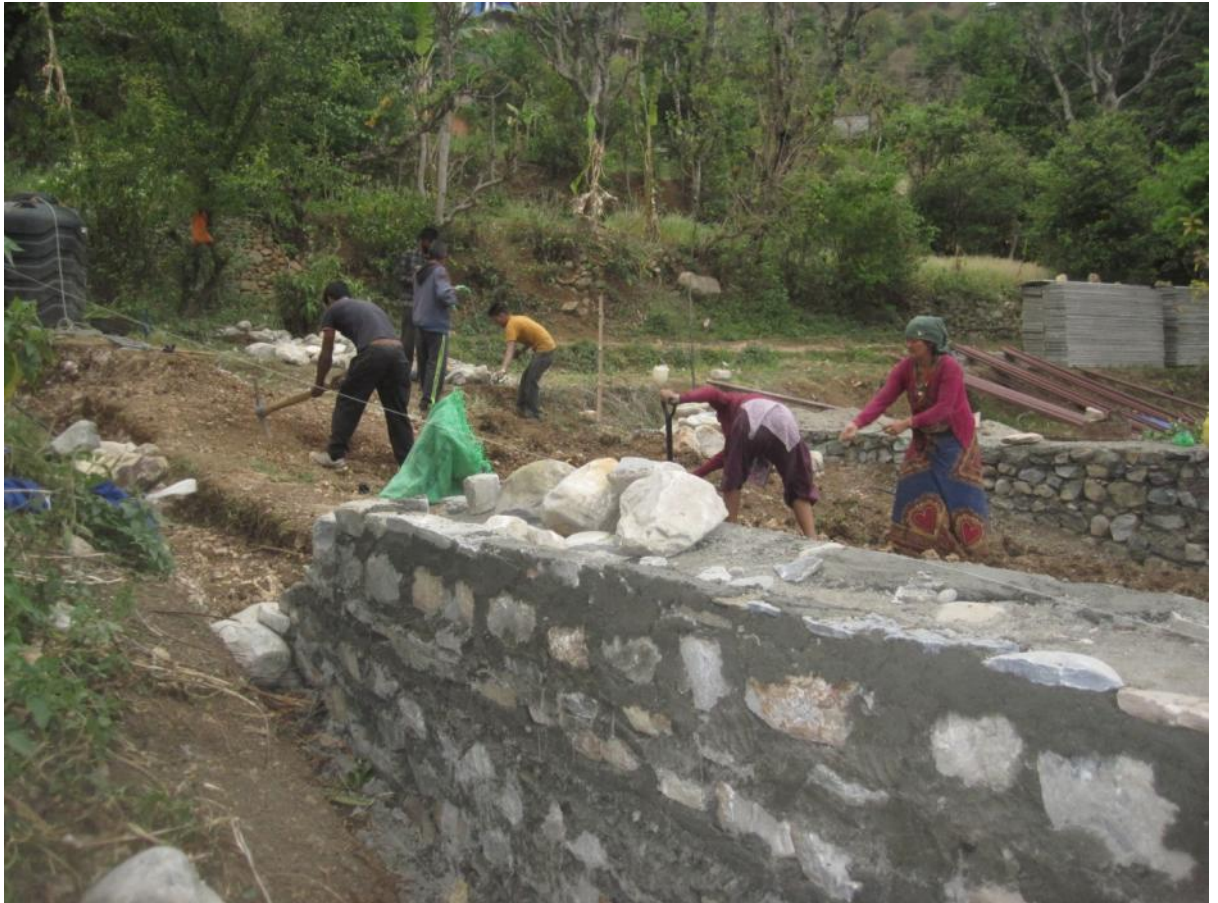
Figure 6: Excavation for leveling and earth filling on constructed wall
