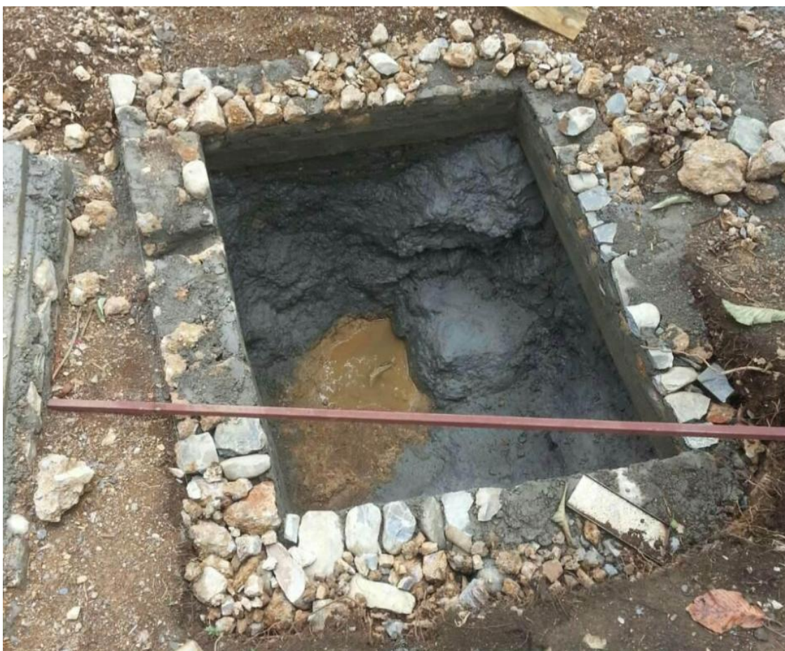
Figure 20: Excavation for Septic tank and stone masonry wall work
