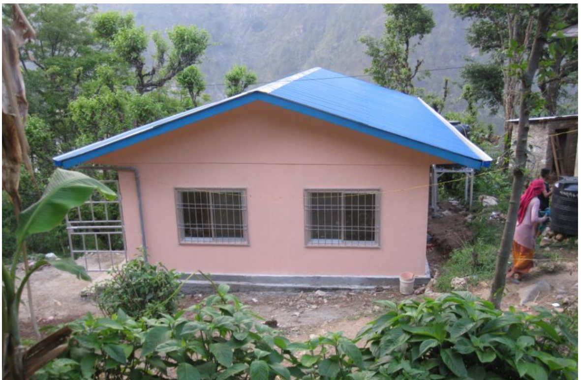
Figure 26: From road view of completion building
