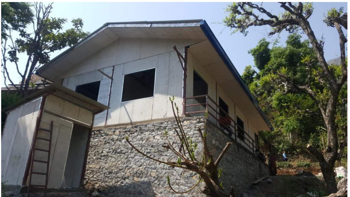
Figure 18: False ceiling installation & toilet roofing installation
