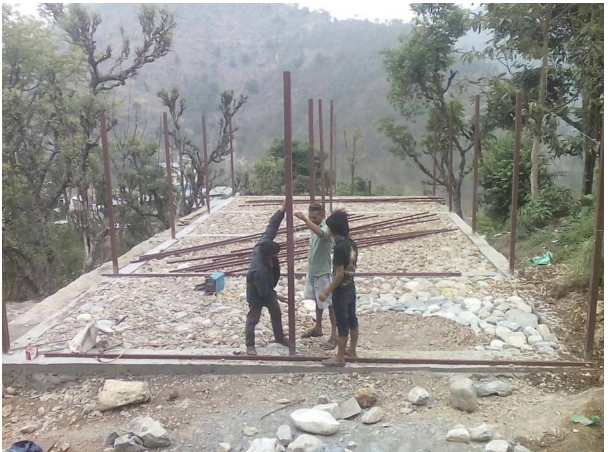
Figure 14: Post leveling for truss installation
