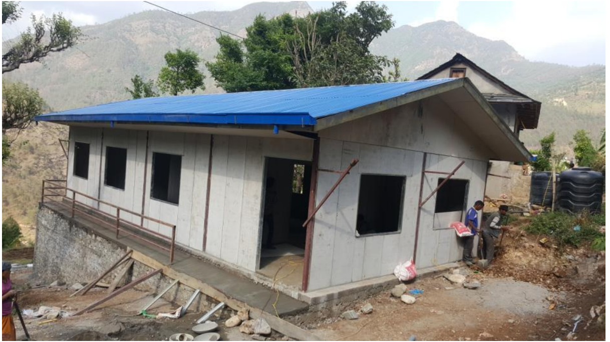
Figure 17: Color CGI sheet & gutter installation
