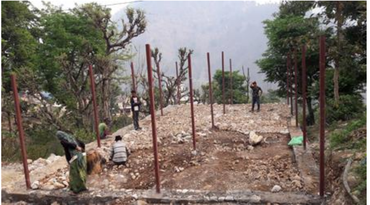
Figure 9: Post erection for truss
