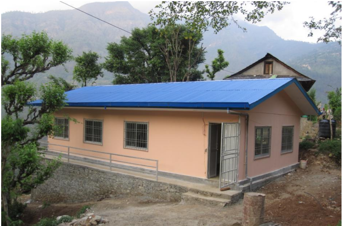
Figure 25: Completion of exterior paint
