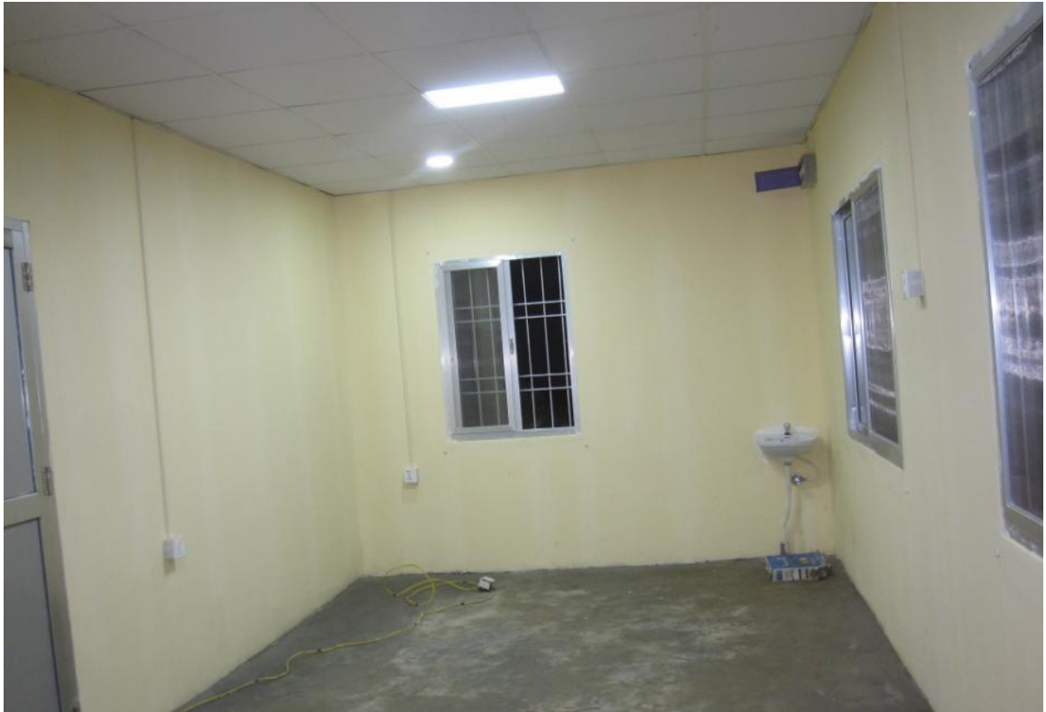
Figure 23: Completion of inner false ceiling, wall paint and electrical
