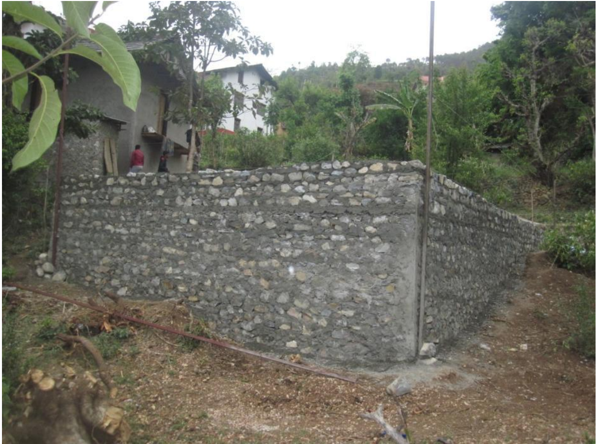
Figure 7: Stone masonry wall completion
