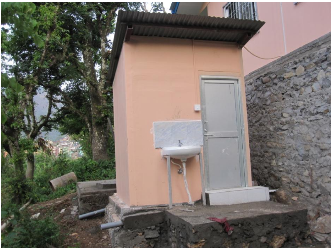
Figure 22: Completion of toilet
