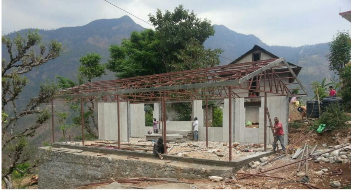
Figure 16: Truss & Prefab board installation
