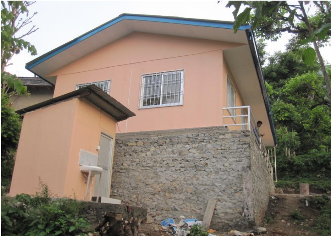
Figure 27: Back side view of building
