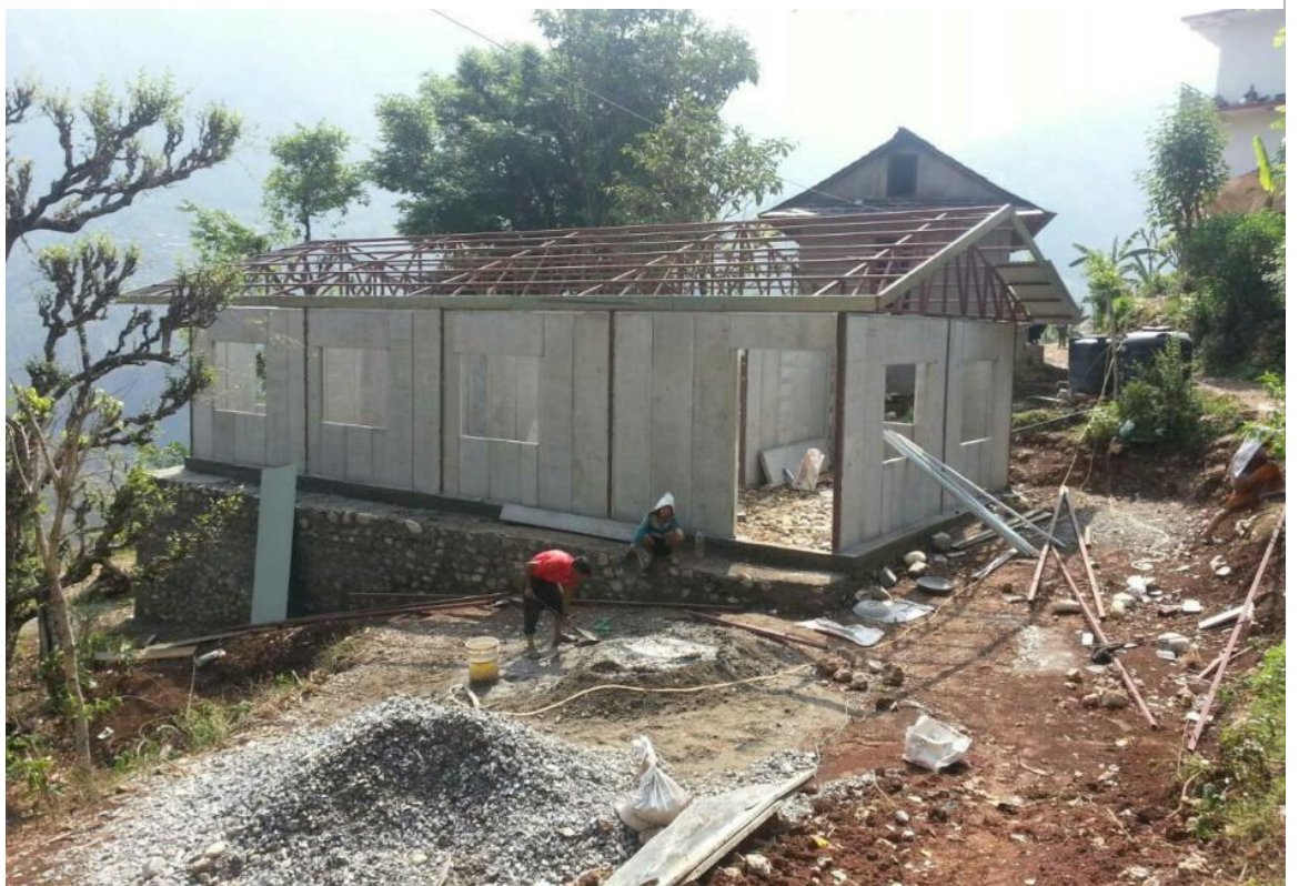
Figure 16: Truss & Prefab board installation
