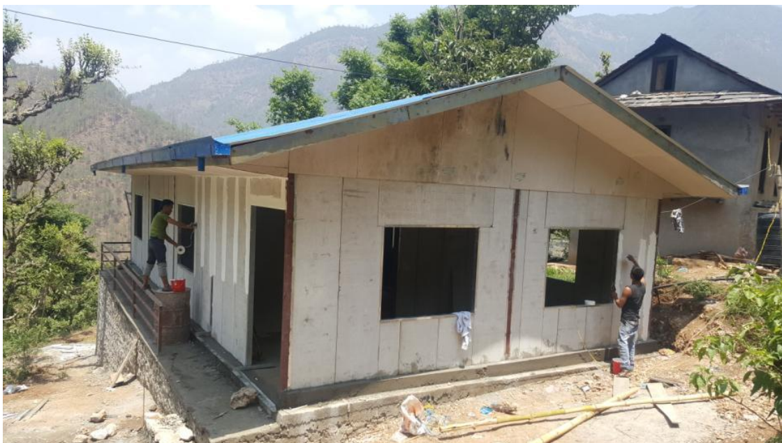
Figure 19: Tapping and putting on wall gap for paint
