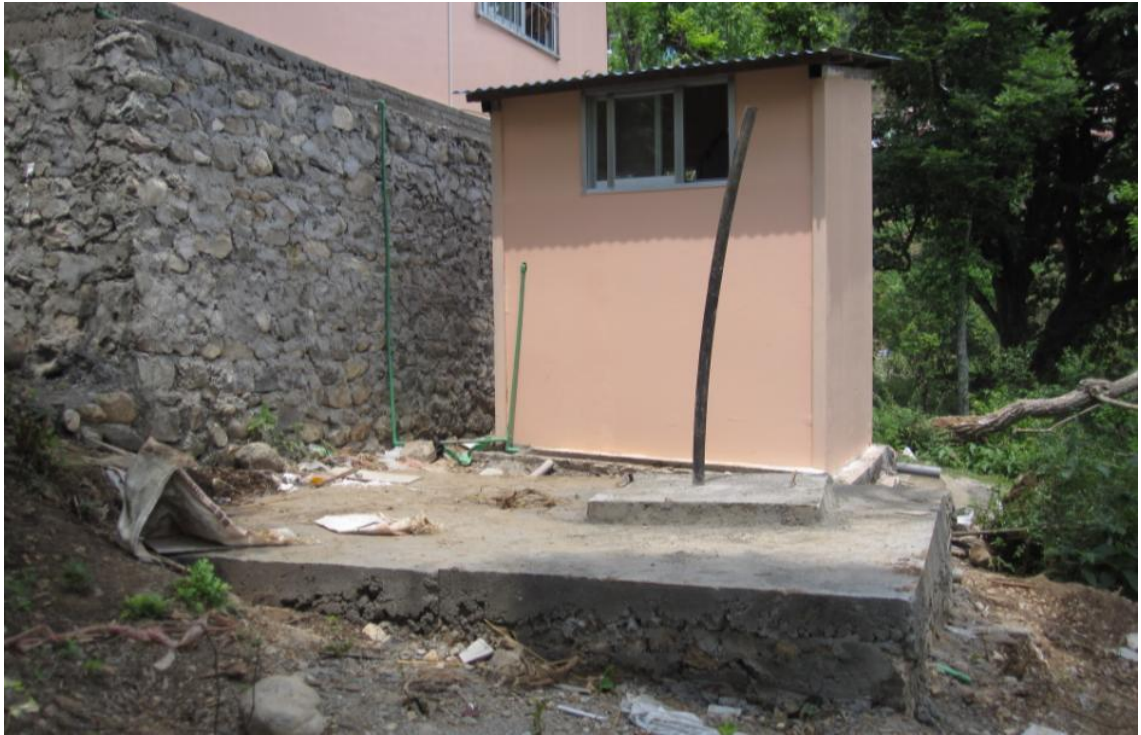
Figure 21: Completion of septic tank
