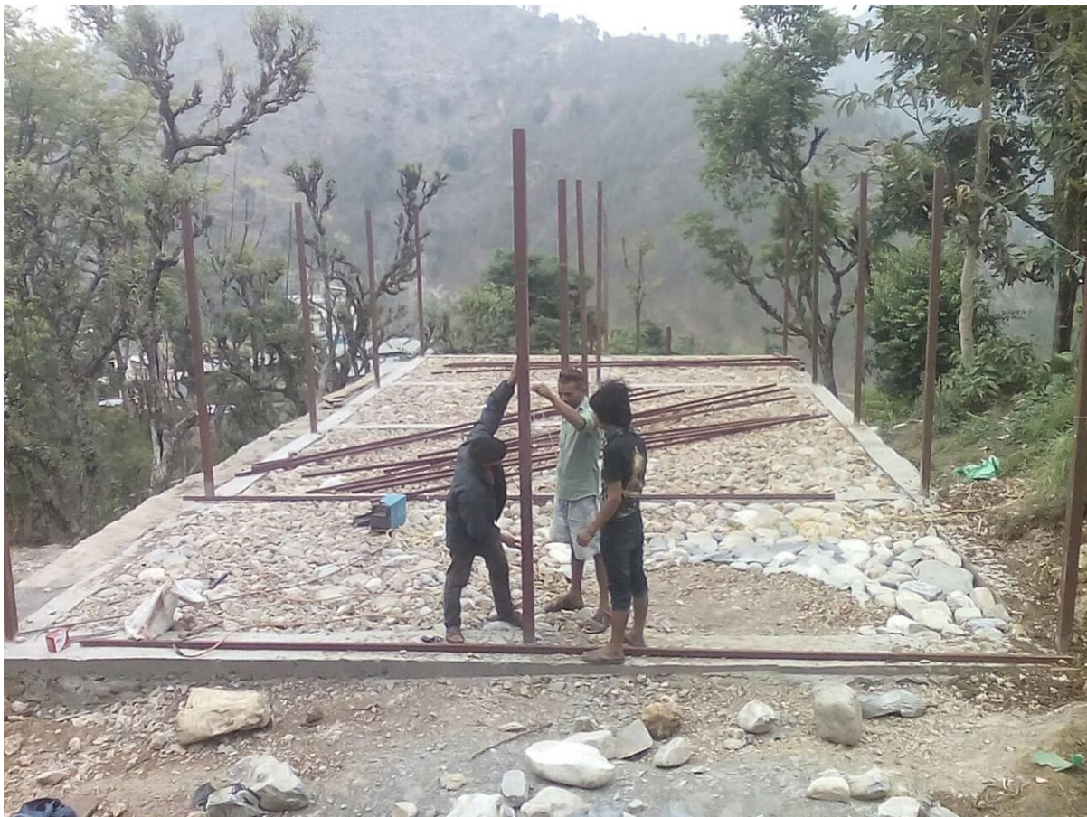
Figure 14: Post leveling for truss installation
