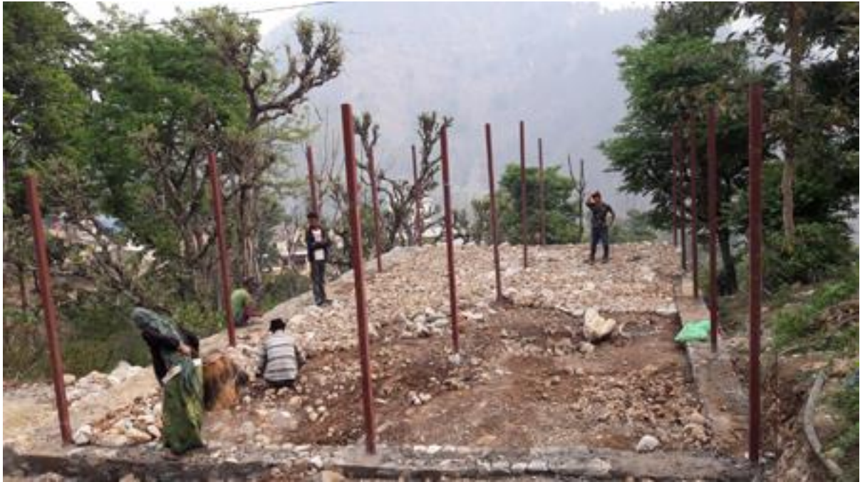
Figure 9: Post erection for truss
