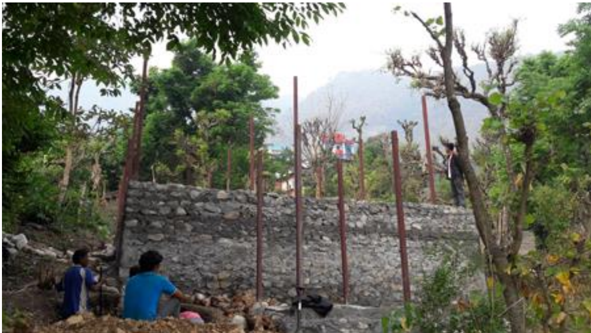
Figure 12: Toilet foundation, RCC & post erection and Septic tank excavation
