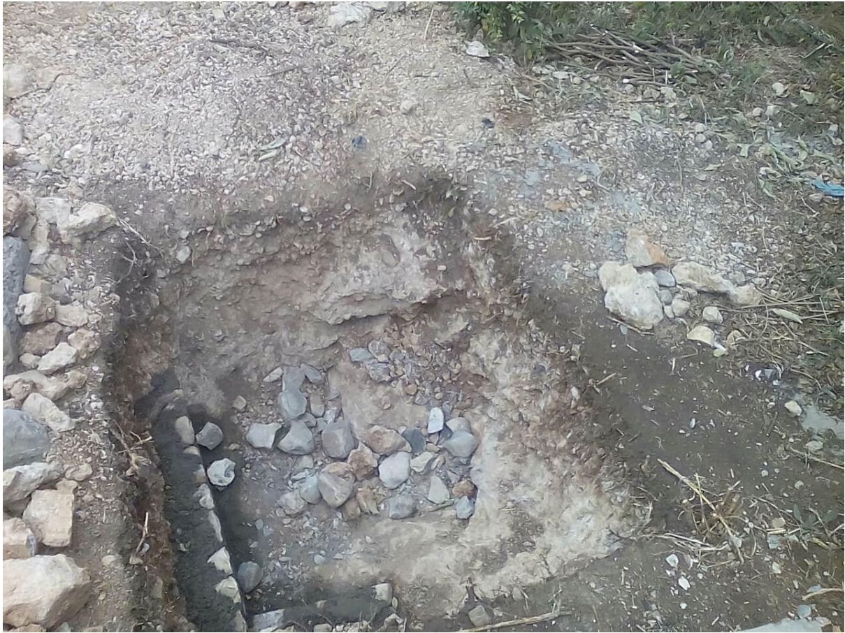
Figure 15: Excavation for Septic tank and stone masonry wall work
