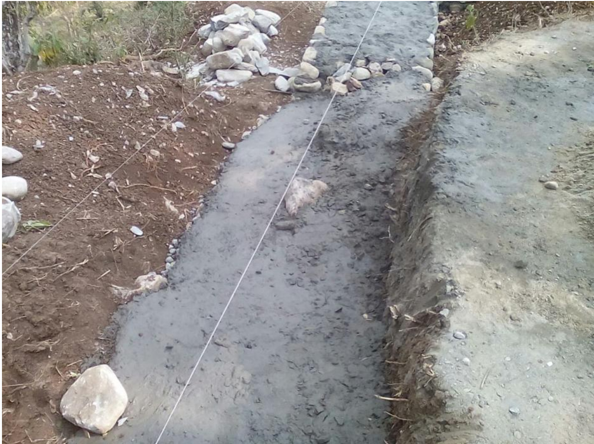
Figure 4: PCC work on foundation after stone soling
