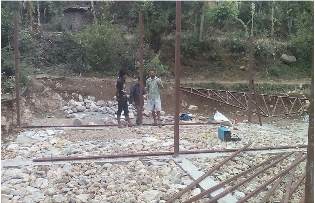
Figure 13: Completion of RCC work and preparation for truss installation
