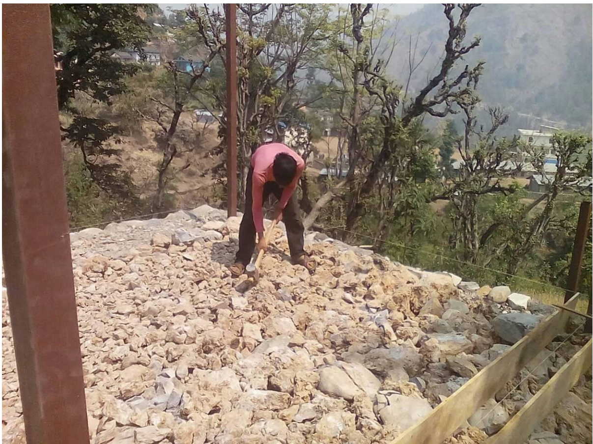
Figure 10: Compaction of soling with hammering
