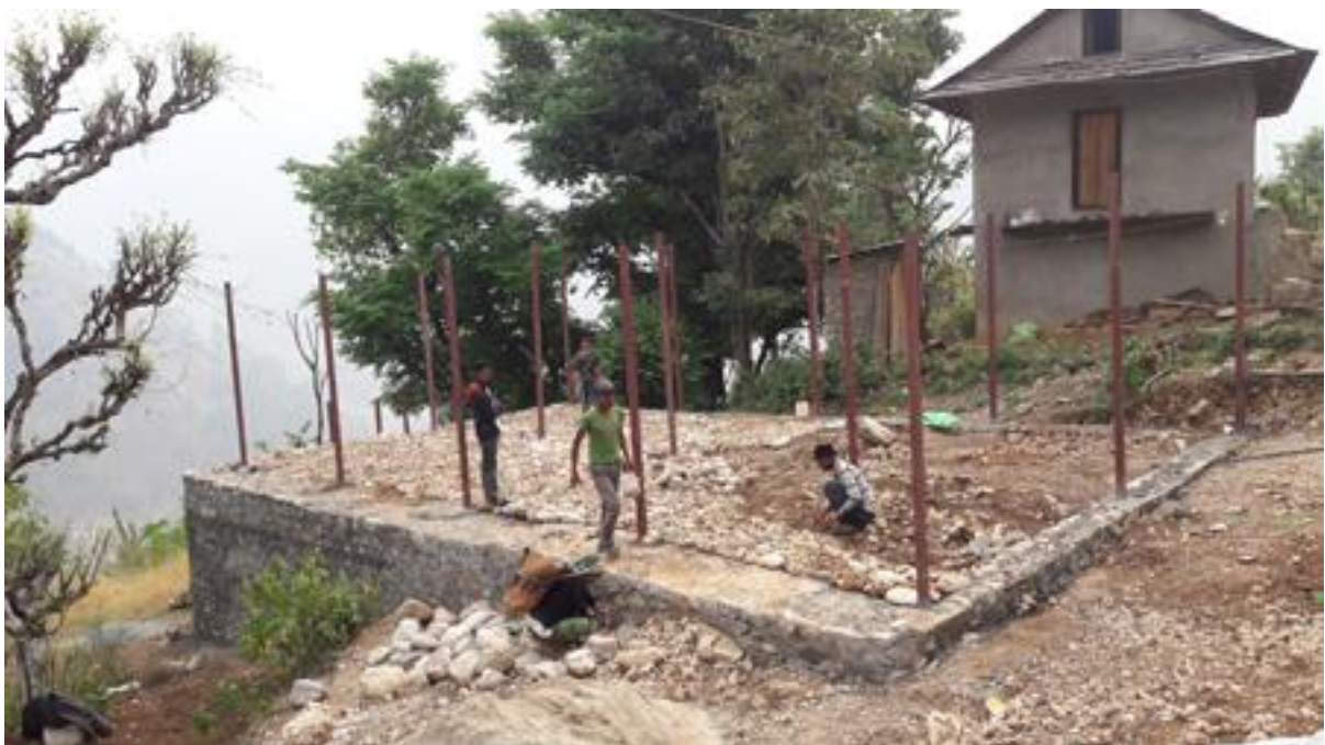
Figure 8: After completion foundation post erection and stone soling for PCC flooring
