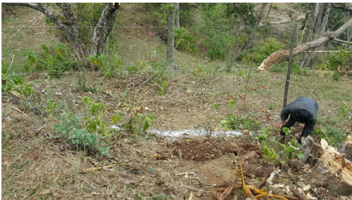
Figure 3: Land layout and side clearance by cutting tree
