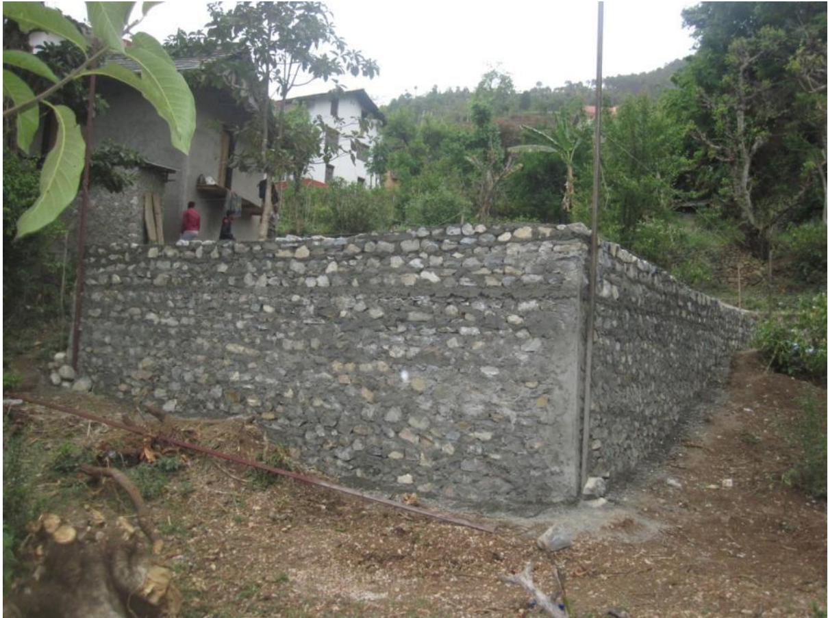
Figure 7: Stone masonry wall completion
