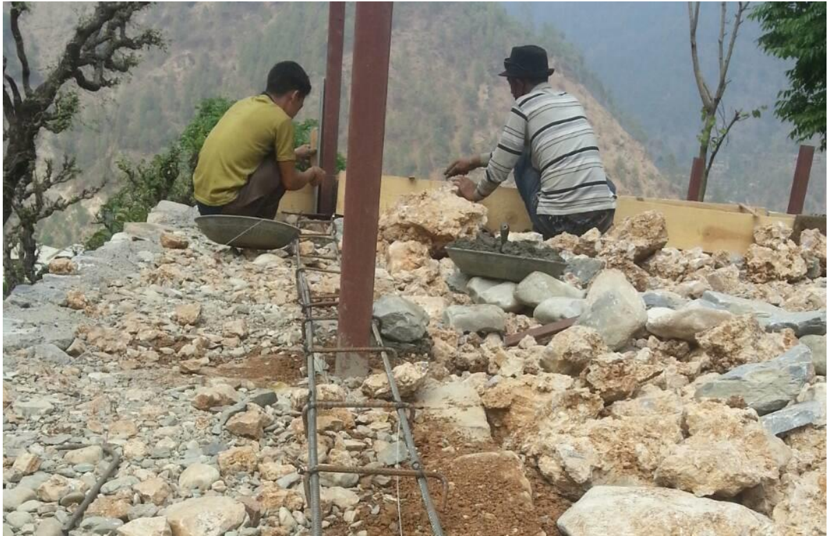
Figure 11: Reinforcement binding and formwork for RCC work
