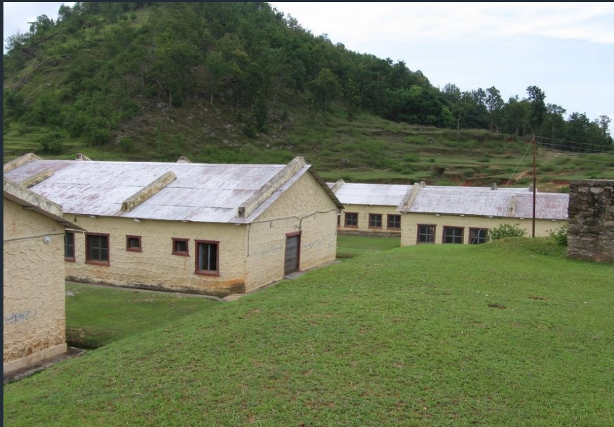
Bayalpata Hospital that Nyaya is renovating
